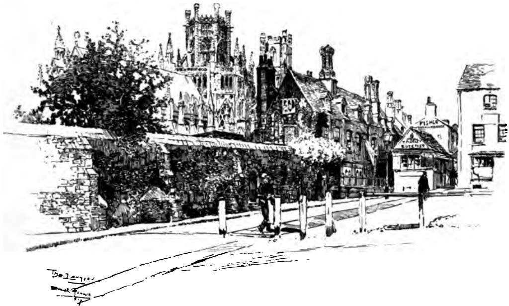
THE LANTERN, FROM THE NORTHEAST.
